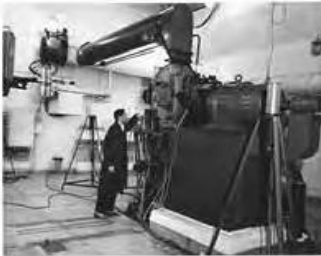
Fig.1. The photo shows the world's first research pulsed fast neutron reactor of periodic operation (IBR).
